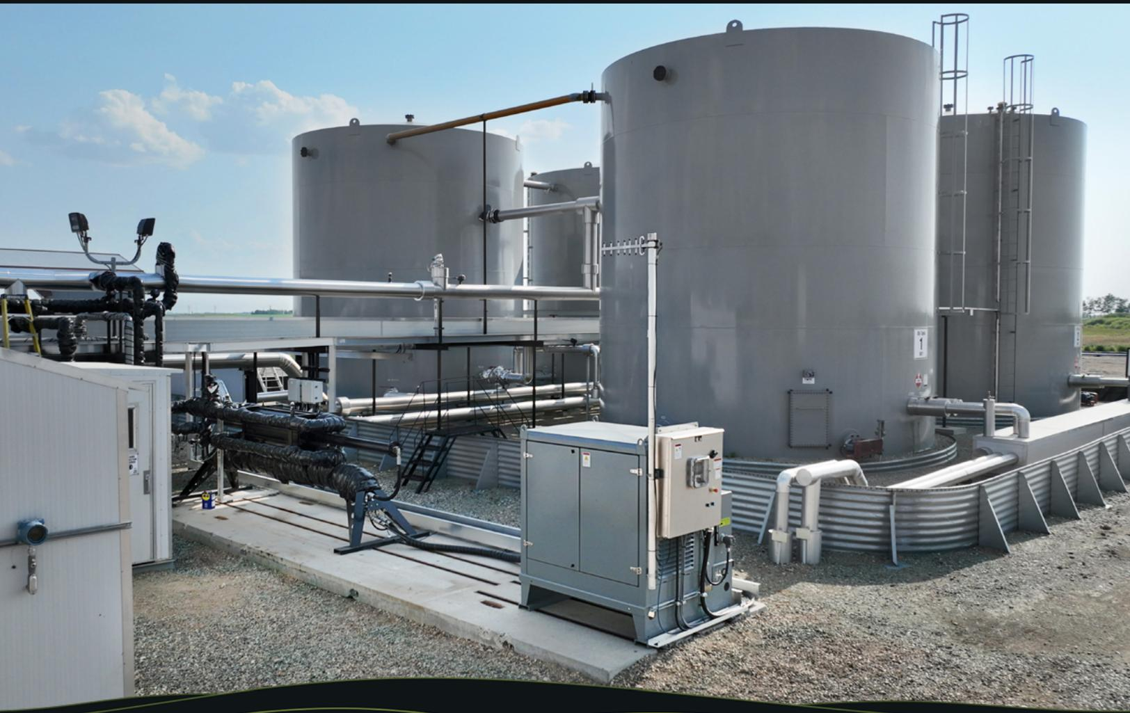
**IJACK VRU** AUTOMATED VAPOR RECOVERY UNIT IS DESIGNED TO REMOVE VAPOR GAS FROM INSIDE TANKS AND VESSELS, ENSURING THAT INTERNAL PRESSURE IS MAINTAINED AT A PRE-SET TARGET LEVEL. BY ENTERING THE MINIMUM AND MAXIMUM TANK/VESSEL PRESSURES, THE VRU AUTOMATICALLY ADJUSTS ITS SPEEDS TO ACHIEVE AND MAINTAIN THE DESIRED PARAMETERS.
